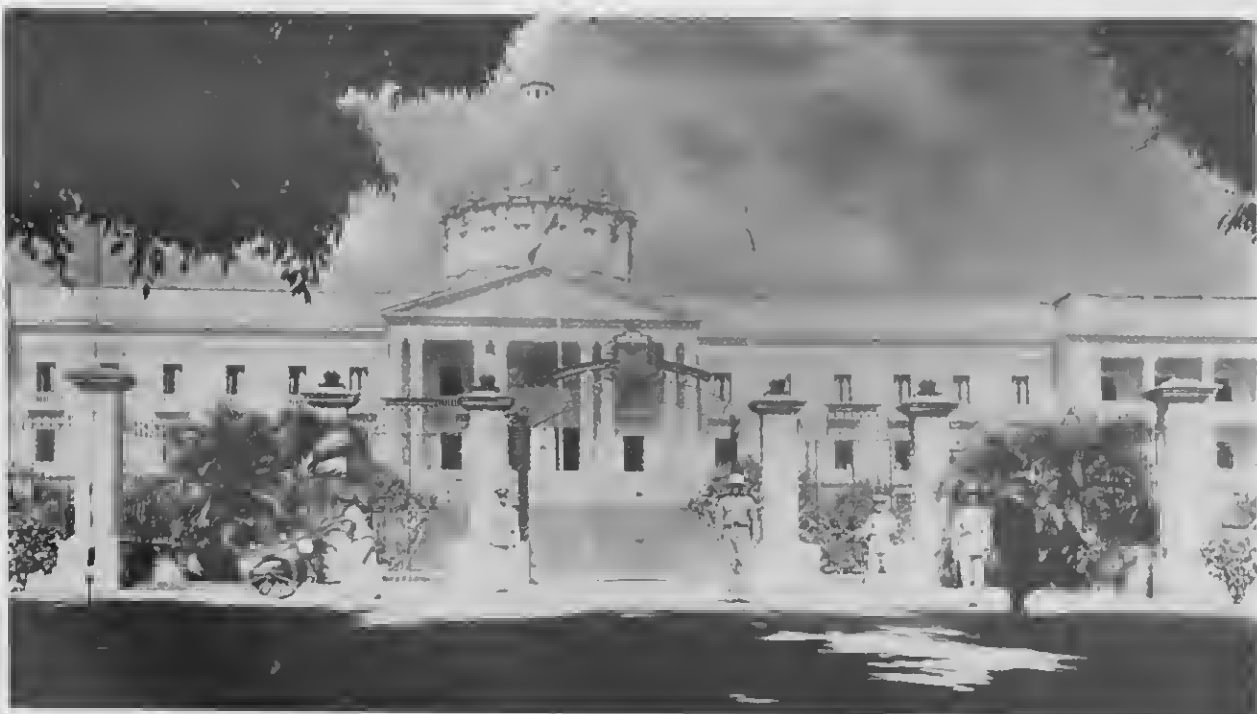
ONE OF the most impressive sights in Ciudad Trujillo is the National Palace. The imposing mansion houses the heart of the city's government. It's design shows the early Spanish influence.
